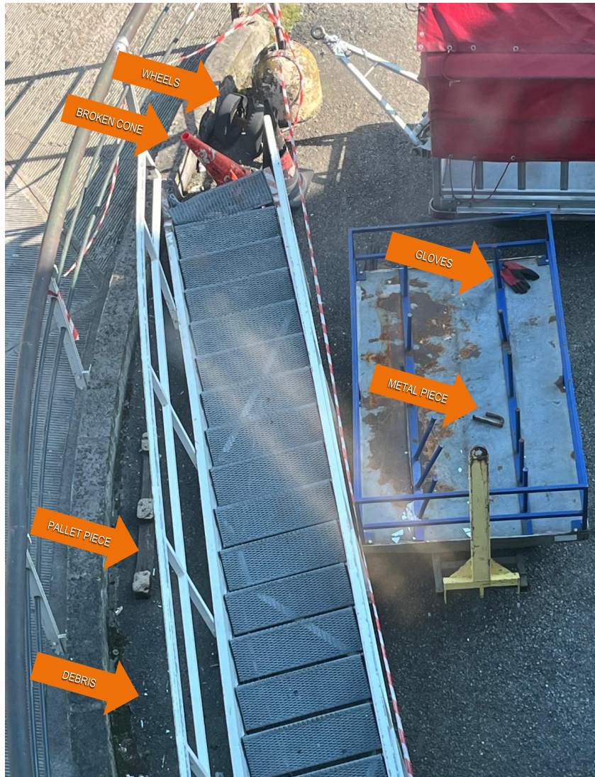
MXP Malpensa Airport – April 30, 2025 – 9:30 am
