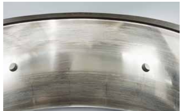
Photo 4.4 Part: Outer ring of Photo 7-4-3 Symptom: Smearing occurs circumferentially on raceway surface Cause: Poor lubrication
