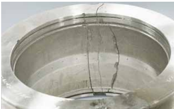
Photo 6.5 Part: Raceway surface of outer ring in Photo 7-6-4 Symptom: Outside surface crack developing on the raceway
